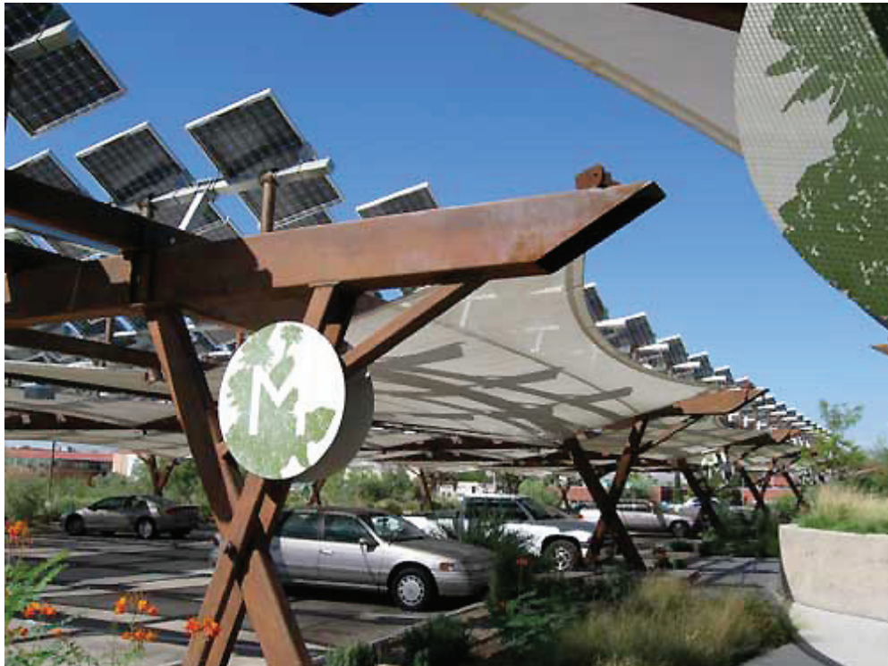
Photovoltaic Panels for Shade: Parking Lot at Springs Preserve, Nevada
