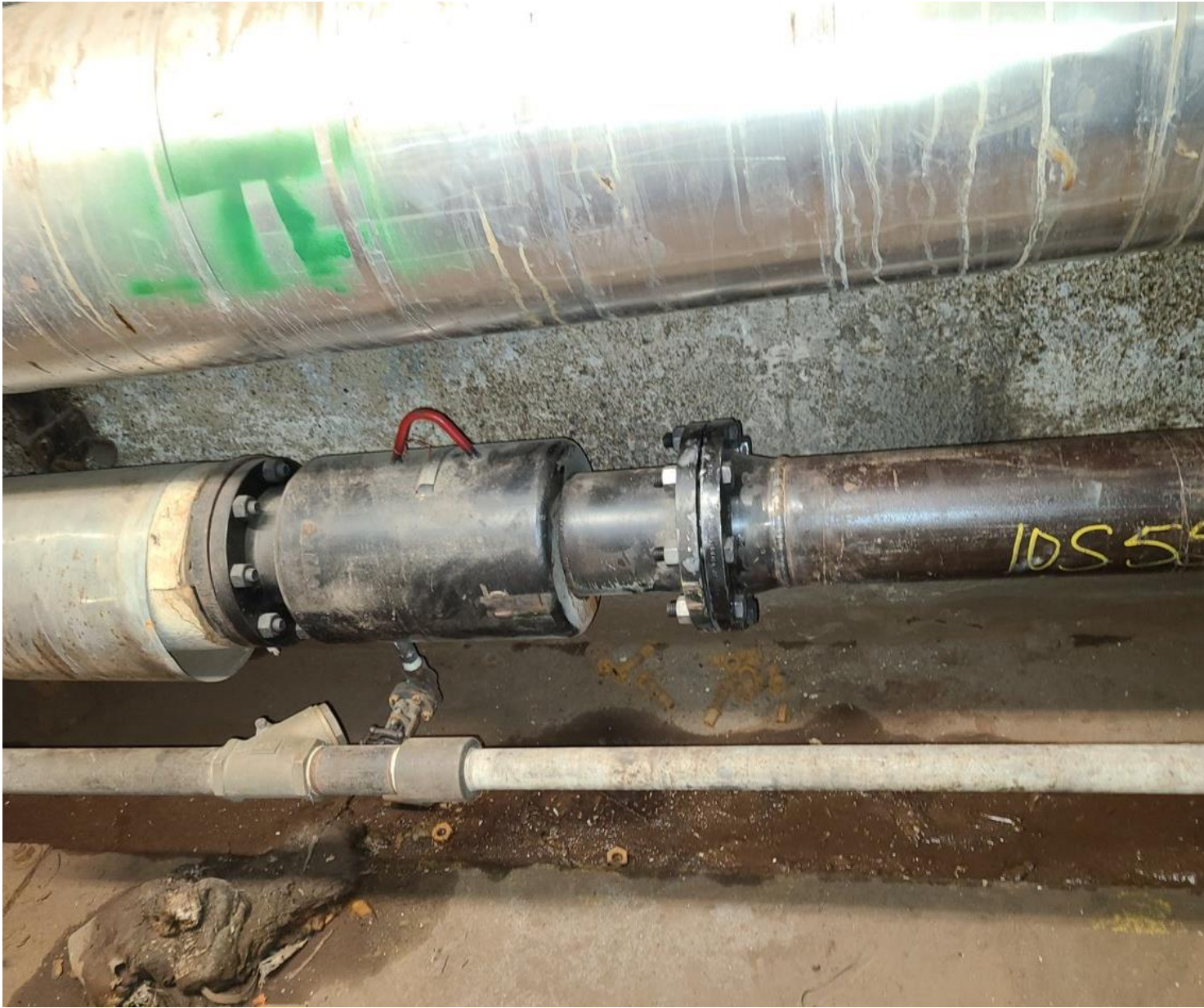
(L) Before: Condensate leak; (R) After: Stop-gap repair measures
