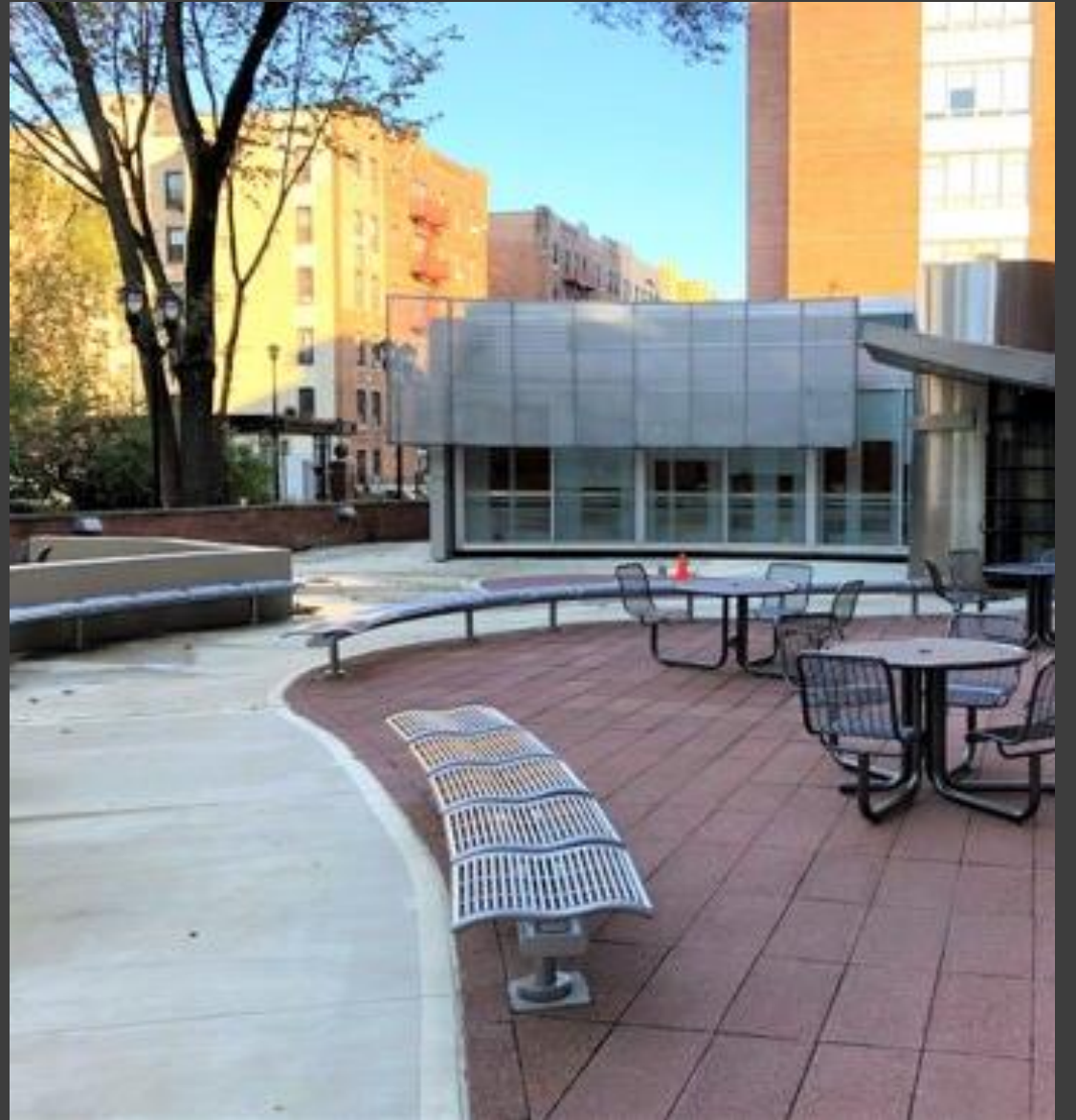
Whitehead Plaza Renovation
