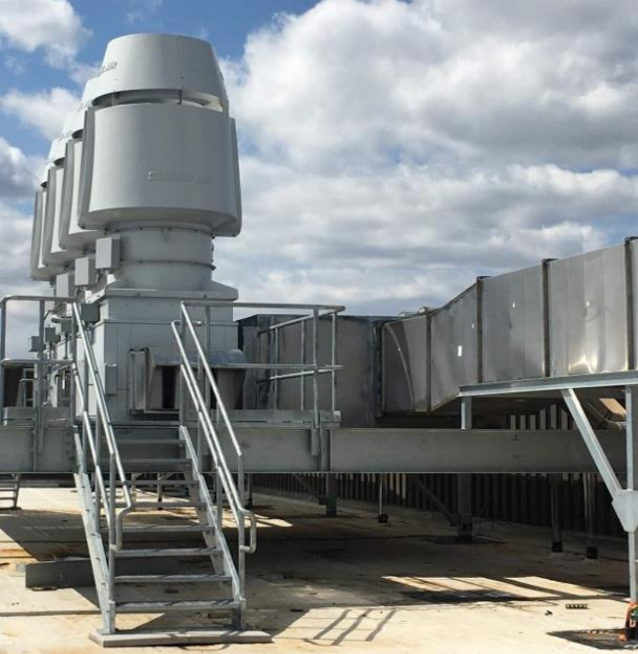
Ingersoll Labs Renovation and Roof Replacement
