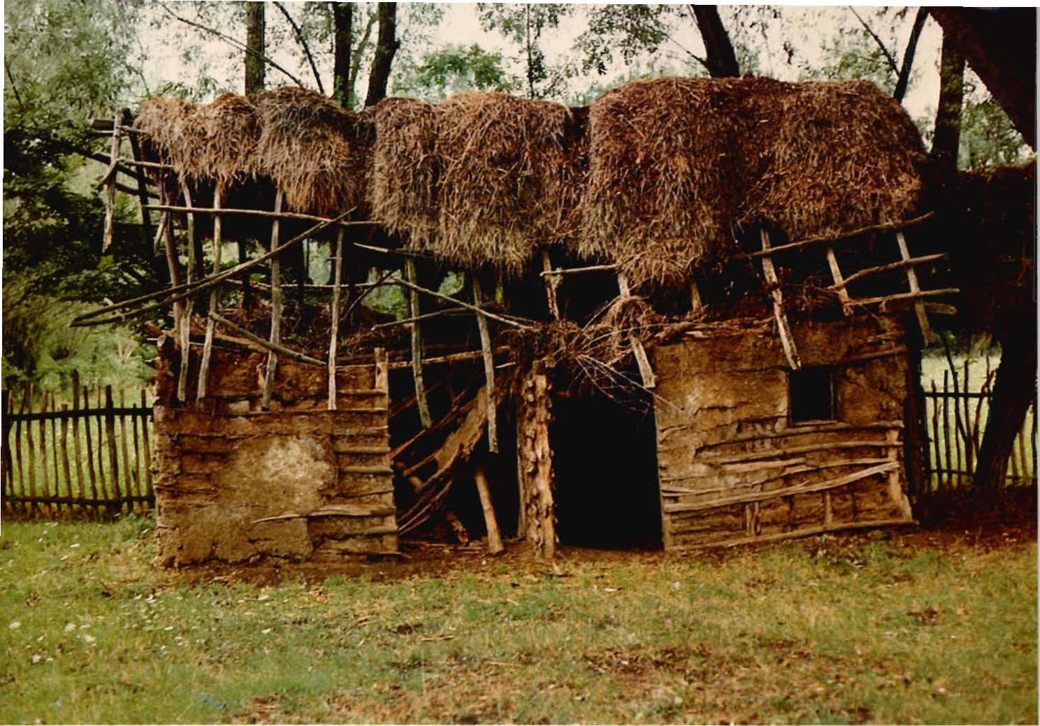
Abandoned wattle and daub house in the vicinity of Jerinin grad in northeastern Serbia. Built some time after World War I, the house has a thatched roof, a western living room with a window and ceiling (right) and an eastern open-roofed chamber. The house is similar to the wattle and daub houses built throughout Europe during later prehistoric times.
