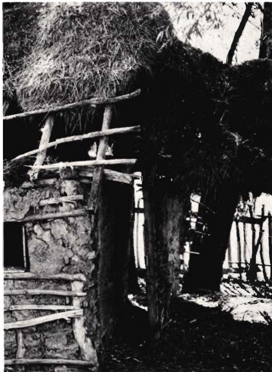
Detail showing the western side of the house and part of the open-walled shed attached to it. Part of the wattle skeleton of the house and the northwestern corner beam are exposed where the daub has flaked off the walls.
