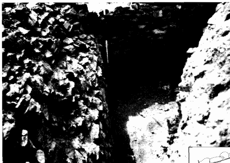
Fig. 48. Interior East corner - wall construction from individual courses of stones separated by a mud seating - Trench 14, Trench 9.
